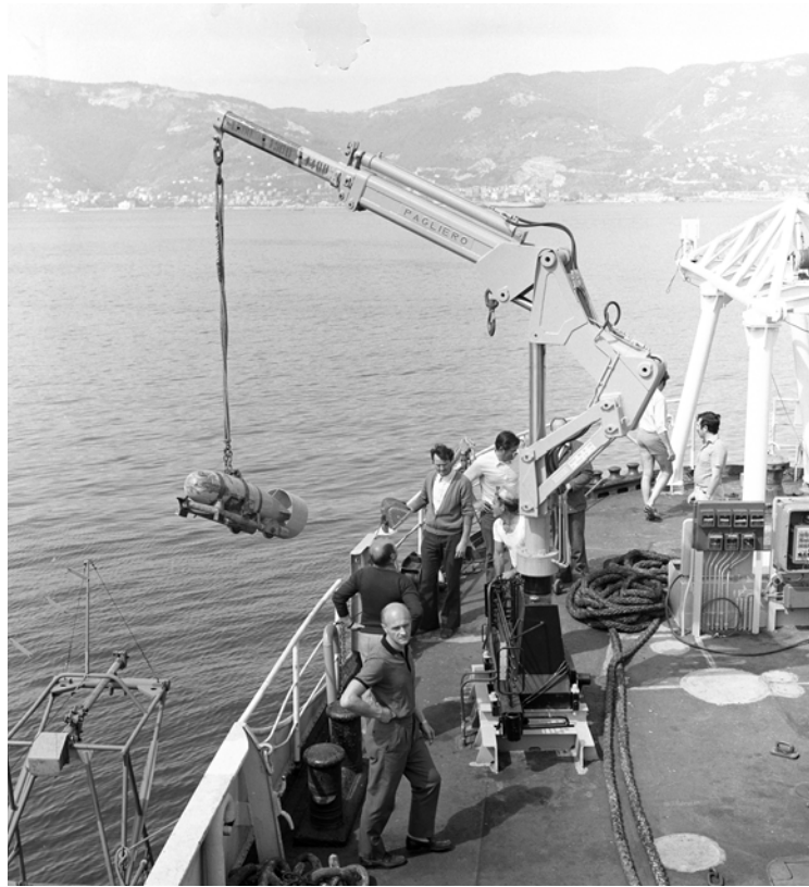
Above: c. 1960s. Crews deploy a towed transducer.
