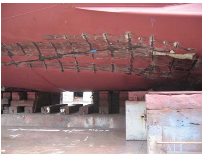
Figure SMO 4 NRV Alliance – underwater hull damage.
