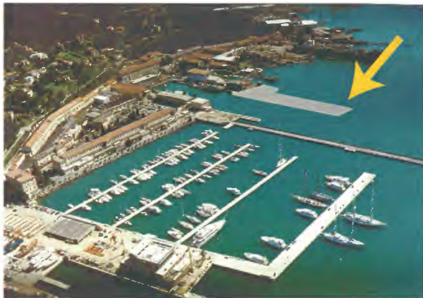
The site of the new pier.
